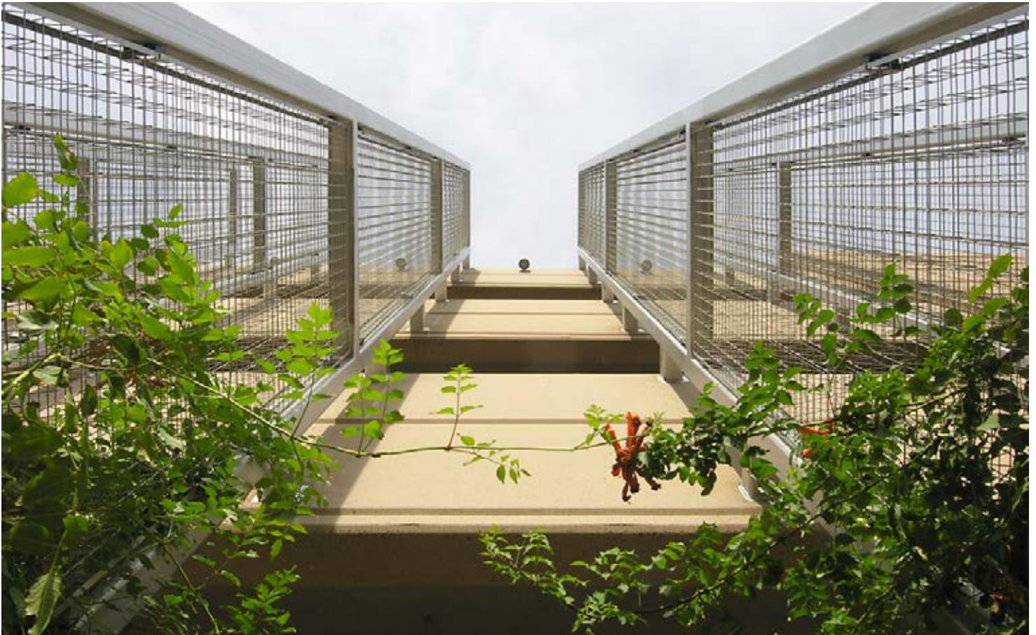
Project: LDS Institute at Arizona State University Parking, Tempe, AZ • Architect: Architekton • Installer: Skyline Steel • GC: Layton Construction
