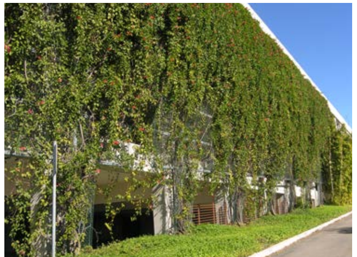
Project: California State University, Fullerton, CA • Architect: AC Martin Partners, Inc.
